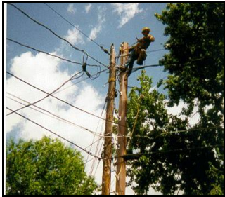
Wood pole replaced by FRP
