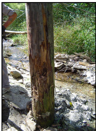
Typical wood pole exposed to extreme moisture
